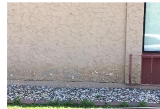
Figure 2 City Hall Exterior Wall
